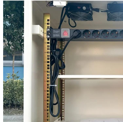
Power source Inverter gasoline generator GEIF55001
